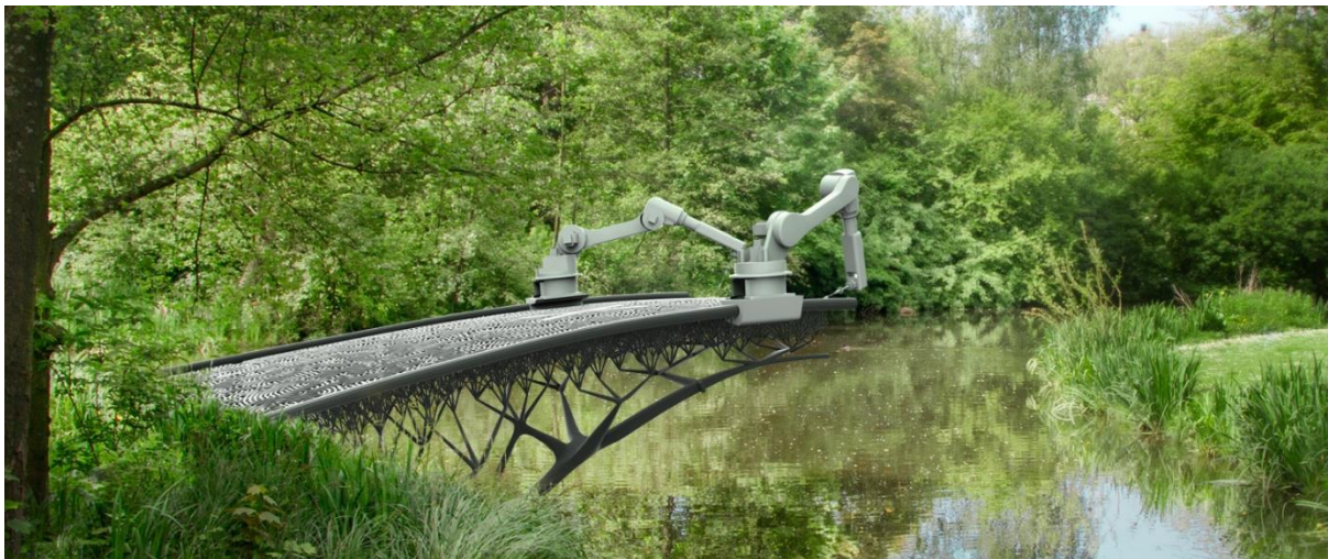
Figure 5 An impression of a 3d-printed bridge that artist and designer Joris Laarman's start-up company MX3D is planning to build in Amsterdam in 2018.
